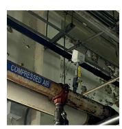
S430 Flow Meter for wet compressed air (insertion type) installation location.
