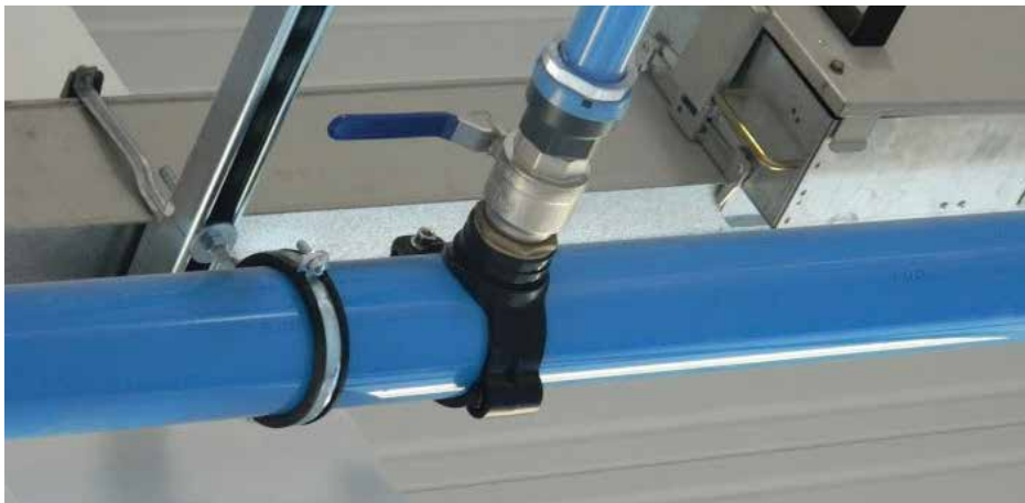
Typical Application for Saddle Branch
