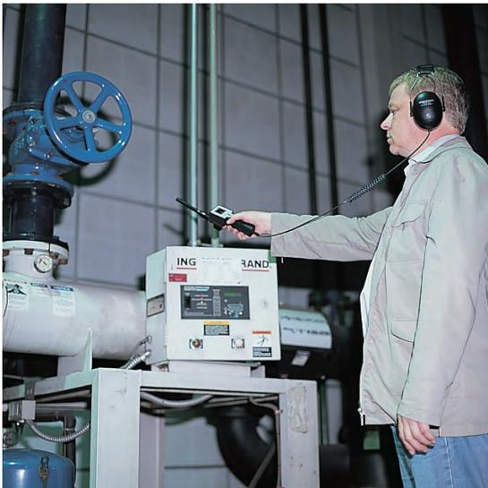
Leak detection with focus tip
