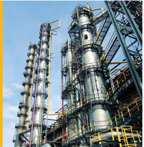
Dryers used to remove moisture from gas, are not always performing as they intend to do, mostly caused by poor maintenance. Dew point measurement acts as an insurance system, monitoring the dryer performance and indicating alarms whenever values are out of valid ranges. As a result it provides:
